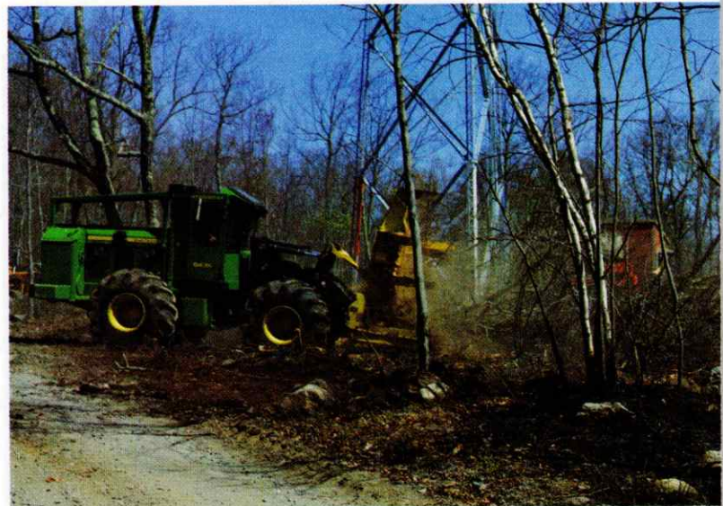
Heavy equipment was brought in to construct a control line.
